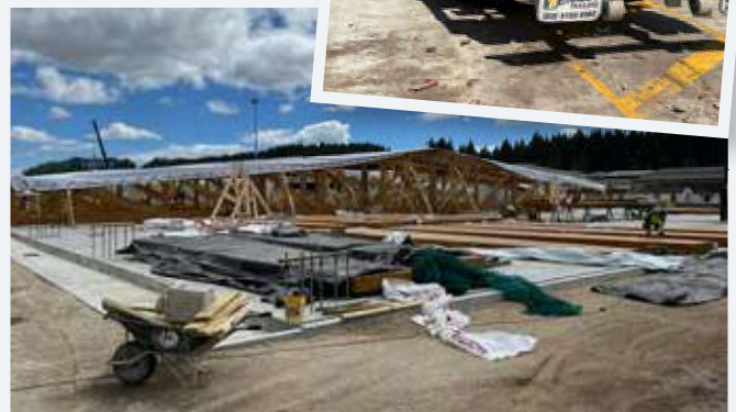
The construction of a new building at Red Stag which uses 65m engineered timber clear span roof trusses (it will be the second largest clear span wooden building in New Zealand).
