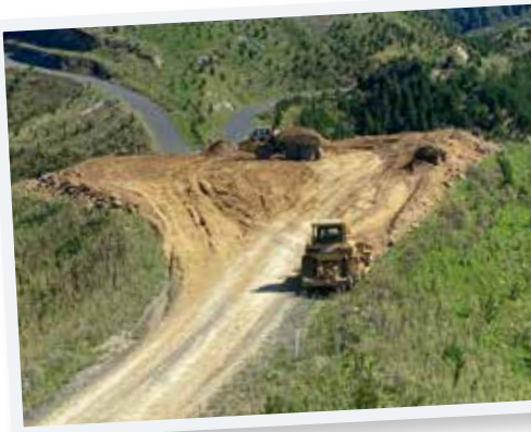
Figure 5 Jilsen: Sometimes the country is too steep to bench and end hauling of skid material is the only option
