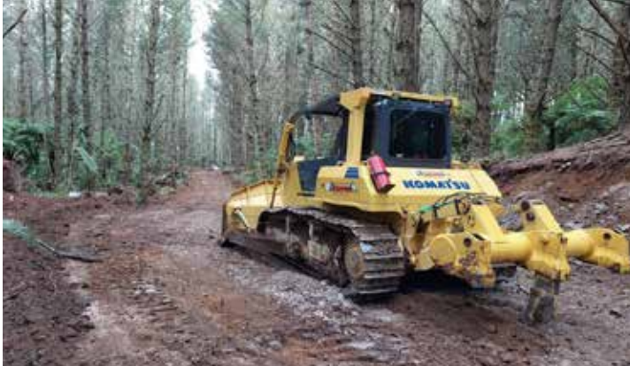
Figure 1 Archer bulldozer forming a new road
