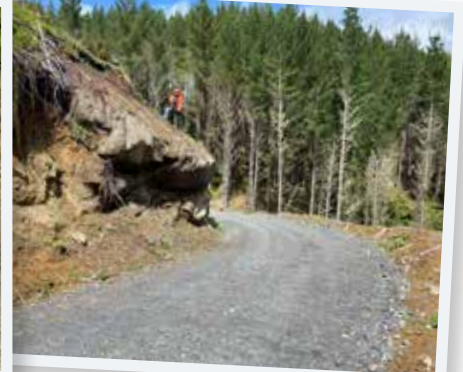
Figure 12 Hand drilling holes for rock blasting can be cheap, quick and effective
