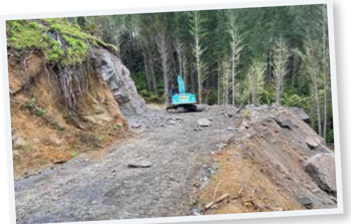
Figure 13 After the blast. Bigger boulders can be used around culverts
