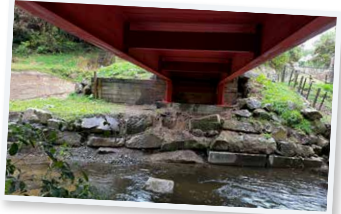
Figure 15 Wagon Road bridge - new cross members and a paint job restored it to a 50max weight limit.
