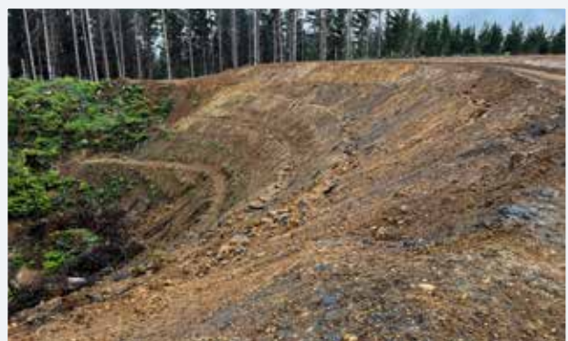
Figure 4 Jilesen: Completed fill benches
