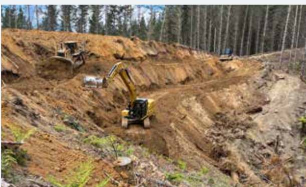
Figure 3 Jilesen: Large skid cut and fill benches using pad foot roller for compaction
