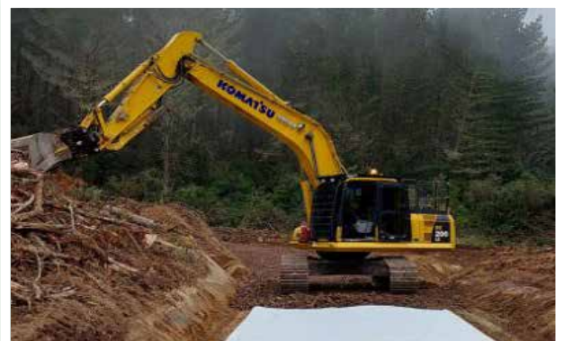
Figure 2 Archer excavator laying Bidum cloth and metal on a formed road
