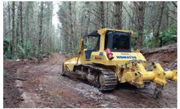
Figure 1 Archer bulldozer forming a new road
