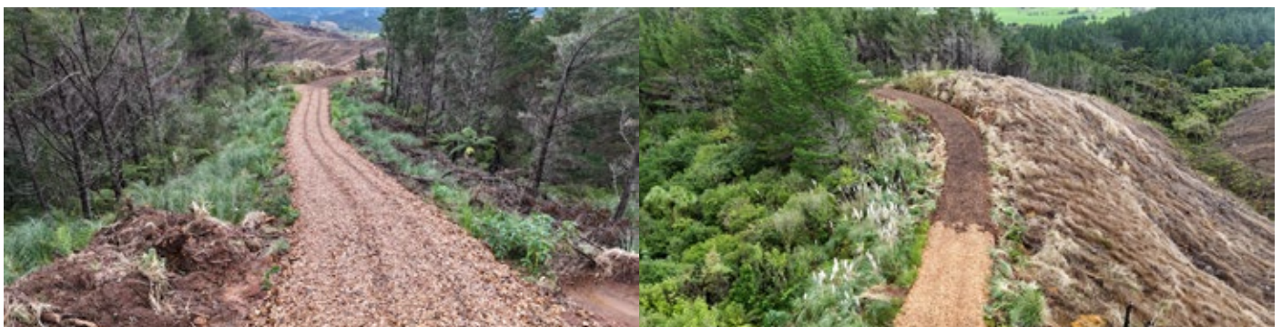
Shred material laid on the road. Shredded binwood has a lighter, cleaner appearance. Shredded slash is the darker material with more bark content.
